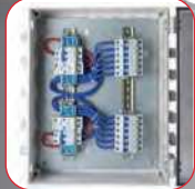
9. DC surge protection
