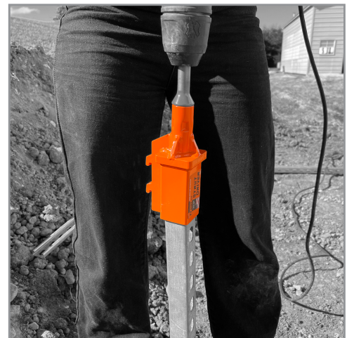
End Receiver for Driving from the Top
