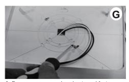
3. Remove necessary knockouts and fasten back plate to j-box.
