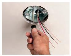
5 Position sled. Tighten screws. Pull cable through installed NM cable connector. Reattach the box to the sled. Attach the fan/fixture bracket with supplied screws.
