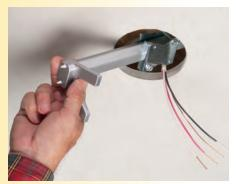
1 Determine location of fan/fixture. Cut a 4-1/16" diameter hole in ceiling. Remove box (only) from the bracket. Loosen screws on sled to enable centering above hole (step 5). Insert bracket through the opening.
