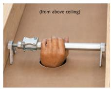
2 Position bracket between joists with "feet" resting on the ceiling. Embed bracket ends in joists by turning the hex bar by hand...
